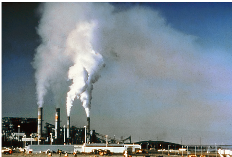
Figure 22.4: A power plant and its emissions before emission control equipment was added. (8)
