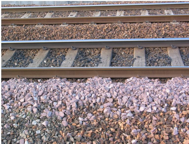
Figure 4.25: Crushed quartzite is sometimes placed under railroad tracks because it is very hard and durable. (24)
