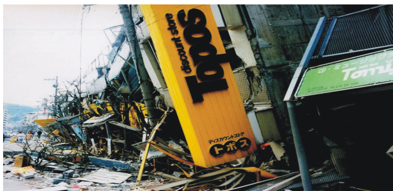
Figure 7.32: Destruction in Kobe, Japan, from the 1995 Great Hanshin Earthquake. (33)
