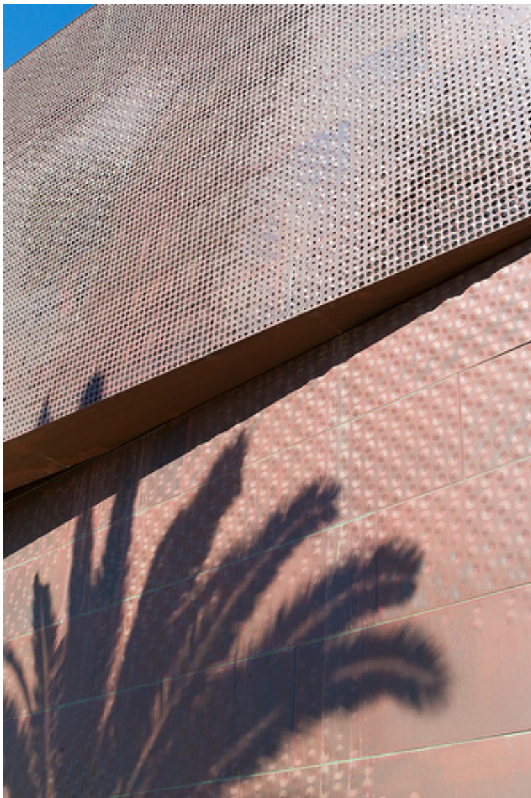
Figure 3.29: The De Young Museum in San Francisco is covered in copper panels. (14)
