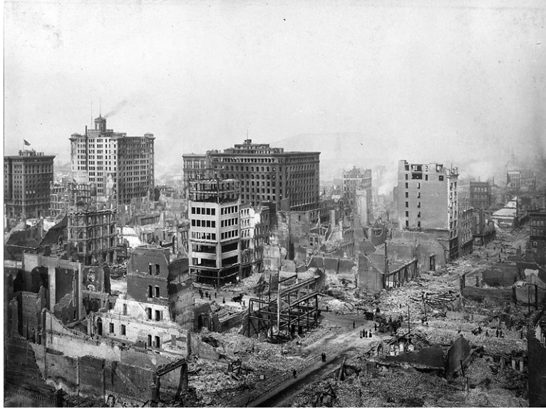
Figure 7.30: Damage after the 1906 San Francisco Earthquake and fire (26)
