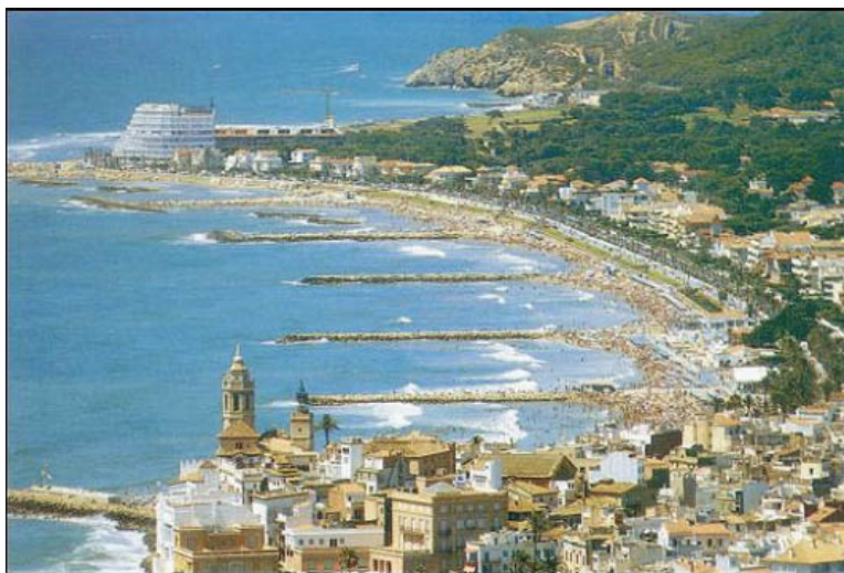
Figure 10.22: Groins are built perpendicular to the shoreline to help keep sand from moving off the beach. (54)
