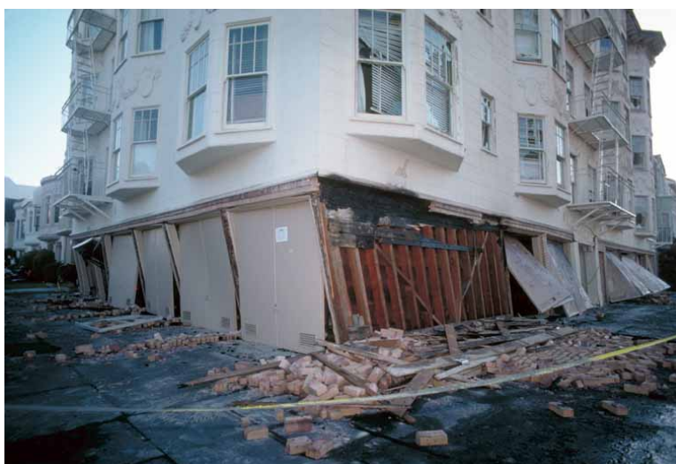
Figure 7.47: The first floor of this San Francisco building is collapsing after the 1989 Loma Prieta earthquake. The building is being held up by the two walls that are not in the photograph and the strength of the upper floors. The two walls that are in view are not strong because they had doors in them. (42)
