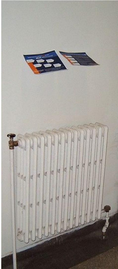
Figure 15.19: Papers being held up by rising air currents above a furnace demonstrate the important principle that warm air rises. (16)
