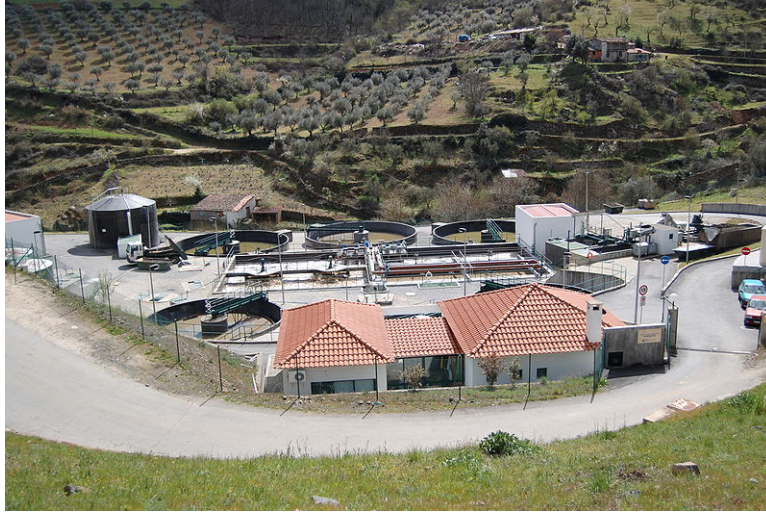
Figure 21.22: Wastewater Treatment: Most wastewater treatment facilities separate contaminants from water by passing wastewater through a series of settlement containers. At each step, solids and particles are separated from water. Chemical and biological agents are also used to remove any remaining impurities. (10)
