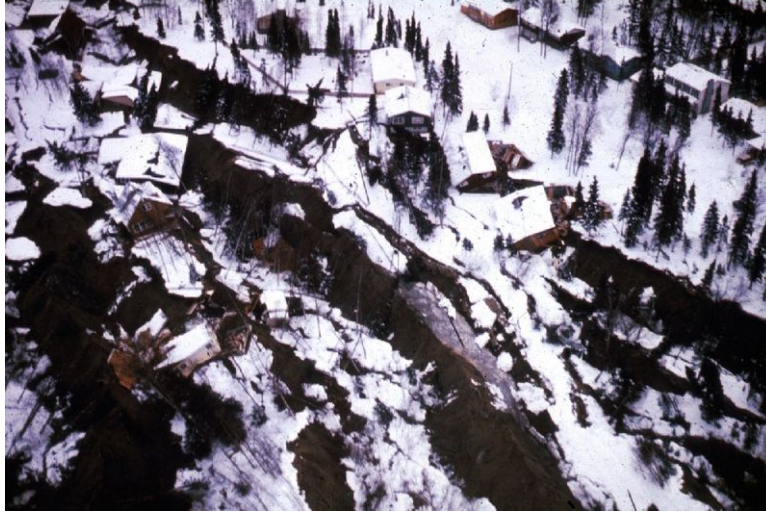
Figure 7.46: A landslide in a neighborhood in Anchorage Alaska after the 1964 Great Alaska earthquake. (29)
